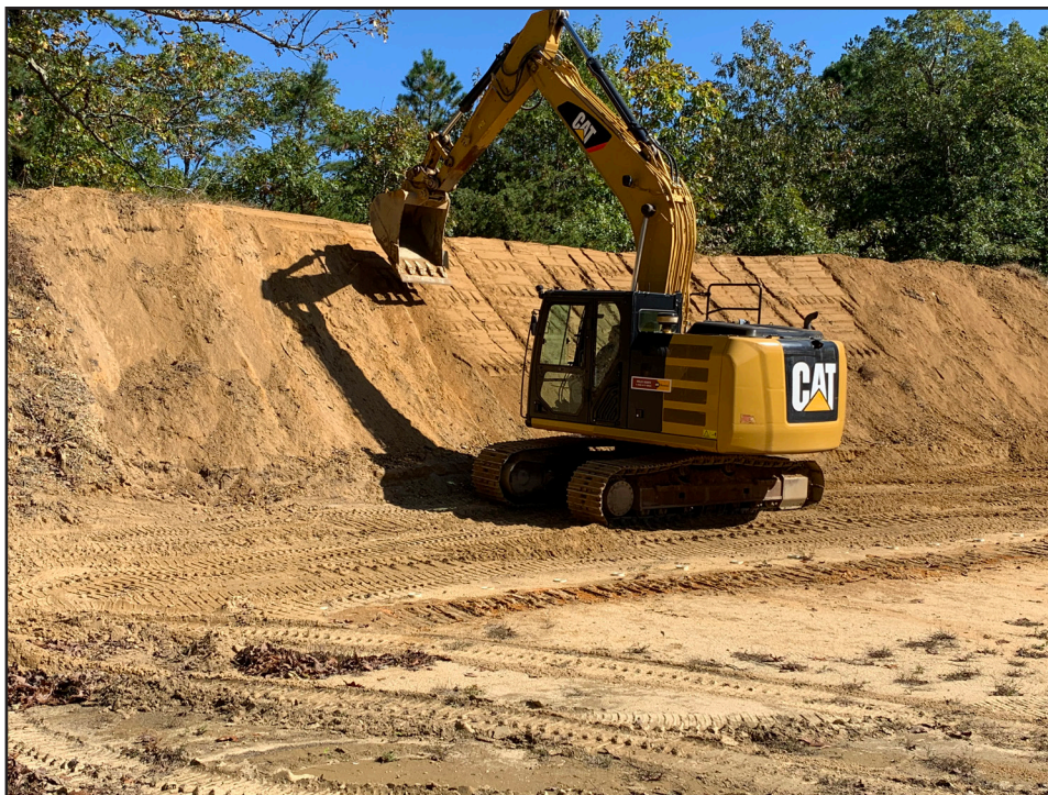
Finishing touches on the 100 yard berm.
